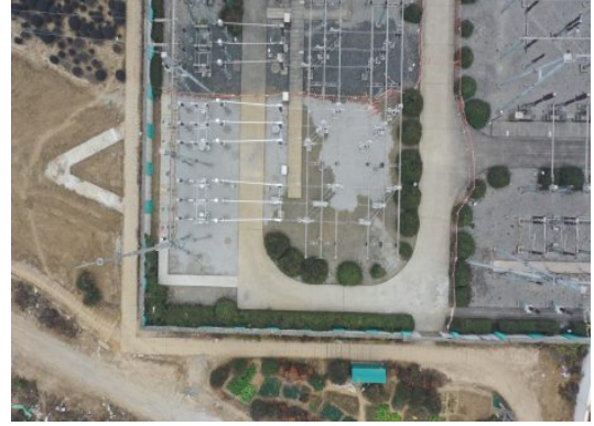
间隔扩建区碎石压盖
