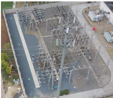
间隔扩建区碎石压盖
