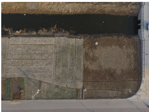
变电站区临时占地复耕 (2020.12.23)
